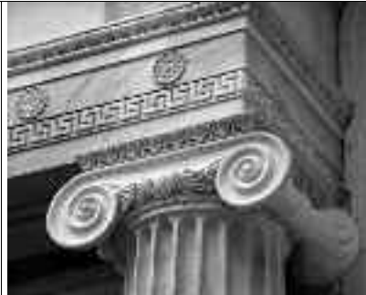
Figure 63 – Greek Key Pattern Around Building
