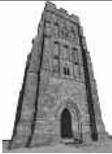
Figure 70 – Remaining Door of Church on Tor Hill, Glastonbury
